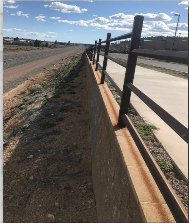
Figure 9: Existing Retaining Wall
