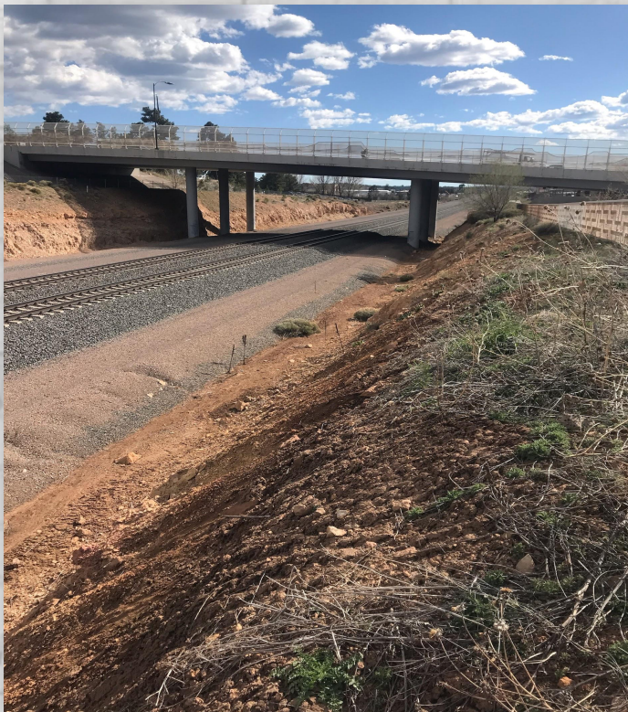
Figure 3: West Wall Location
